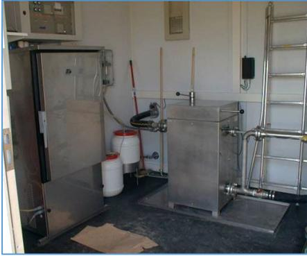
Inside is the gamma spectrometry unit housed in its own tank, surrounded by a strong lead screen protected by a stainless steel casing in which the water pumped from the river enters and leaves – photograph on the left. Ten radionuclides are defined in the recognition software.
