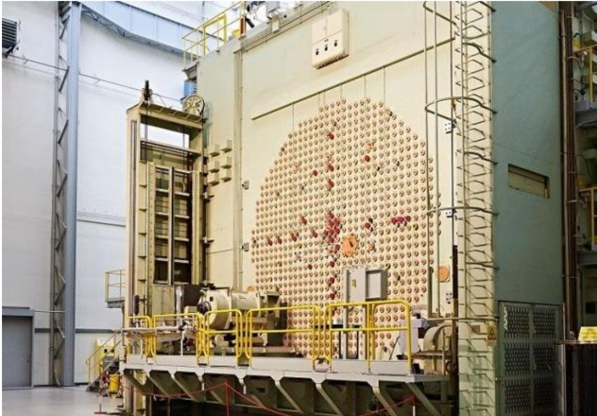
The BR1 is a natural uranium graphite reactor, comparable to the reactors ORNL X-10 (USA) and BEPO (Harwell, UK). The core is composed of a pile of graphite blocks thus forming a cube with ribs of 7 meter. The reactor is air cooled. The fuel is metallic natural uranium with an aluminium cladding. Its design thermal power is 4 MW.
